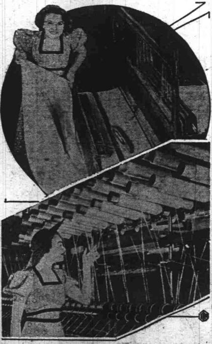
Latest marvel produced by industrial science is glass cloth, now being manufactured at a new plant in Newark, O. Accidental discovery five years ago of a process by which glass thread can be produced led to the new setup and may create another major industry.
