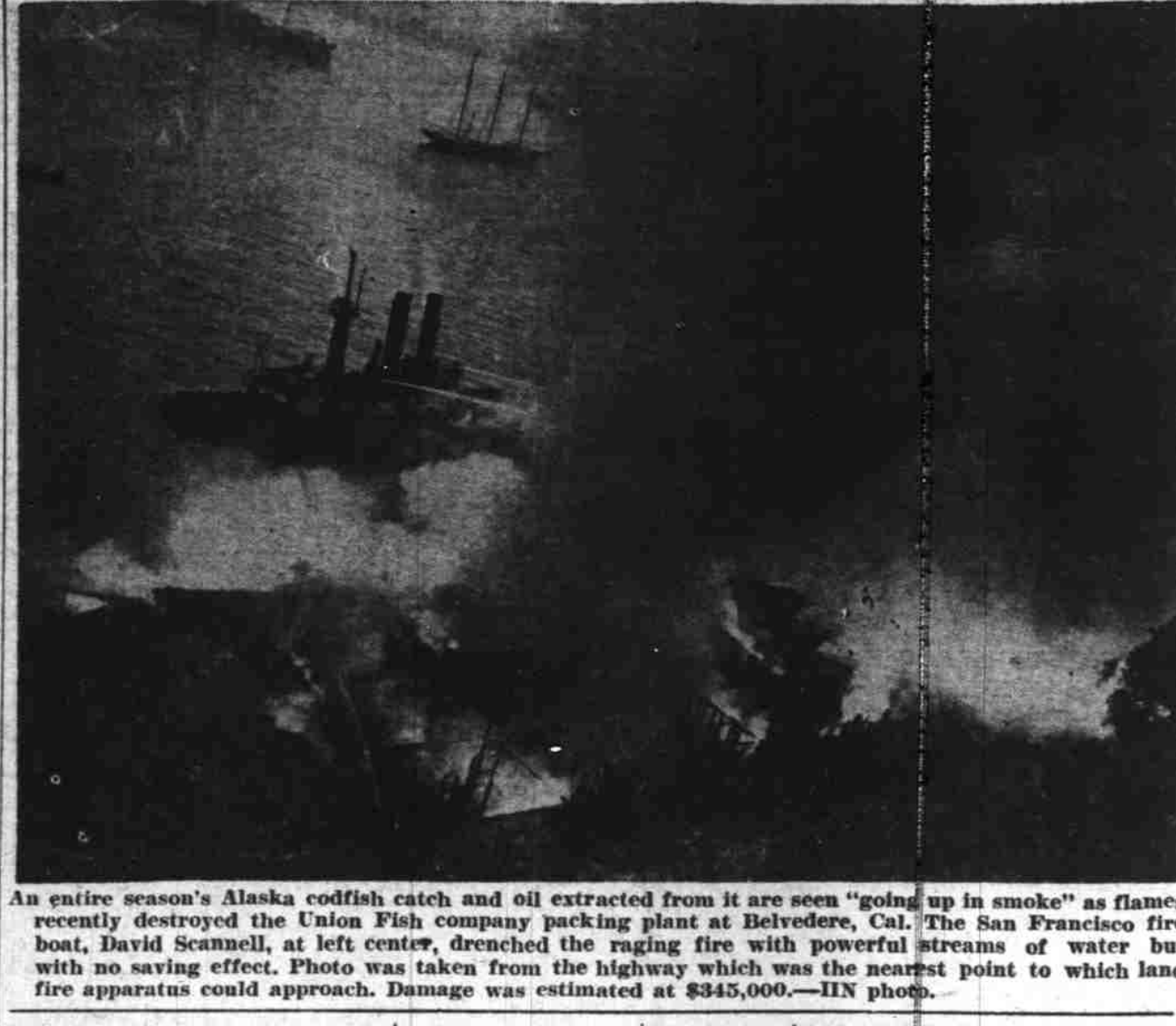
An entire season's Alaska codfish catch and oil extracted from it are seen "going up in smoke" as flames recently destroyed the Union Fish company packing plant at Belvedere, Cal. The San Francisco fire boat, David Scamell, at left center, drenched the raging fire with powerful streams of water but with no saving effect. Photo was taken from the highway which was the nearest point to which land fire apparatus could approach. Damage was estimated at $345,000.—LIN photo.
