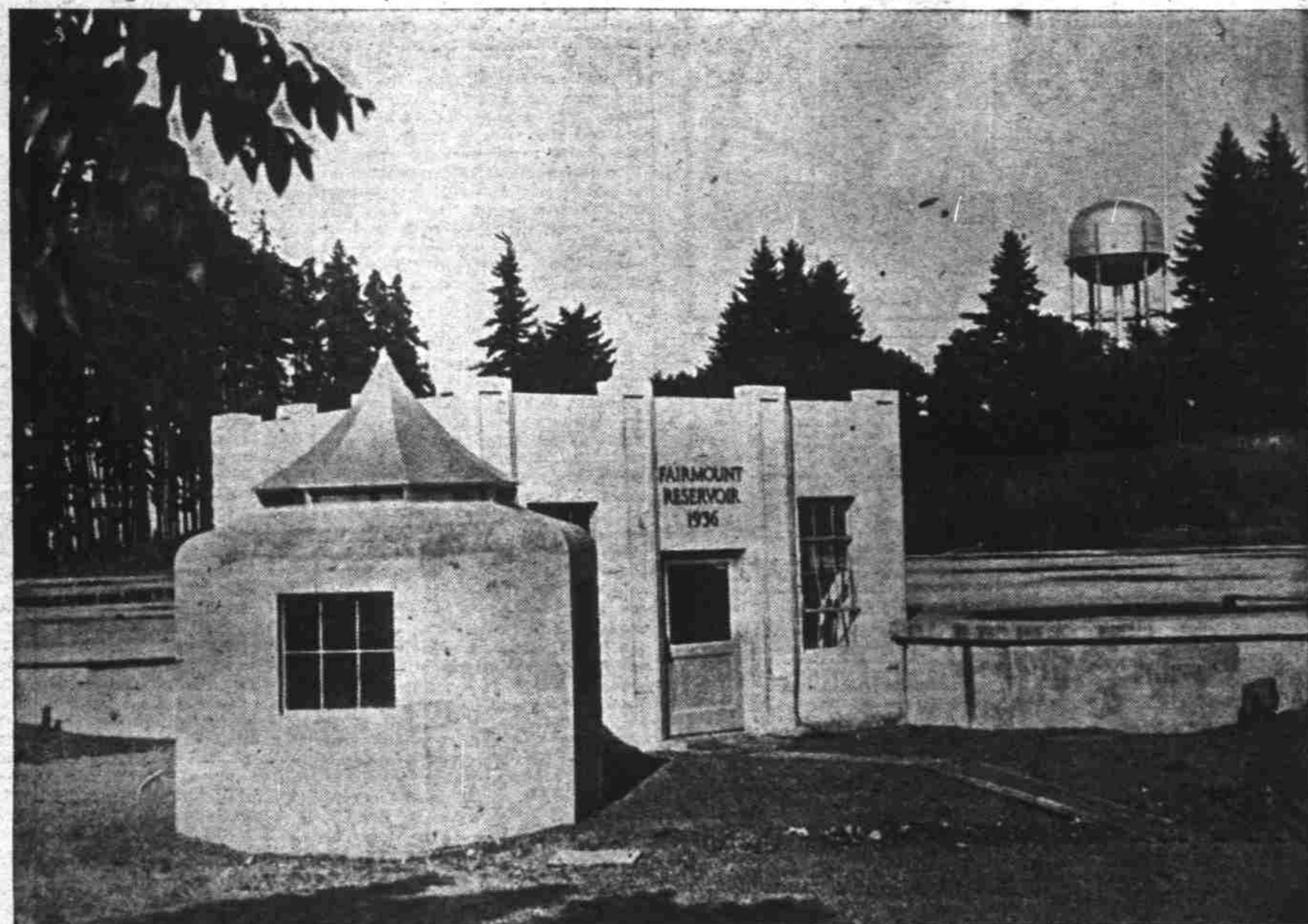
Control house; 10,000,000 gallon reservoir; storage tank in background, on Fairmount hill. Concrete building in foreground is overflow chamber. (Statesman staff photo.)
