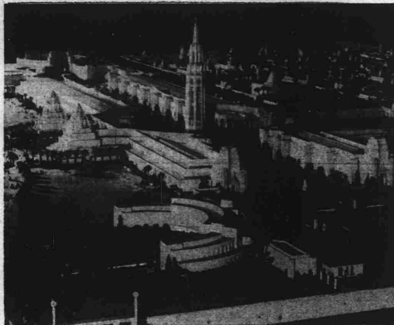
Here is an authentic replica of San Francisco's 1939 Golden Gate International Exposition, now under construction. At left center is the main entrance. In the center is the spire-like tower, which may be used as an airport beacon after the exposition has closed and the man-made island converted into an airport. At upper left automobiles will be parked. The twin buildings to the right foreground will be converted into airplane hangars.—IIN photo.
