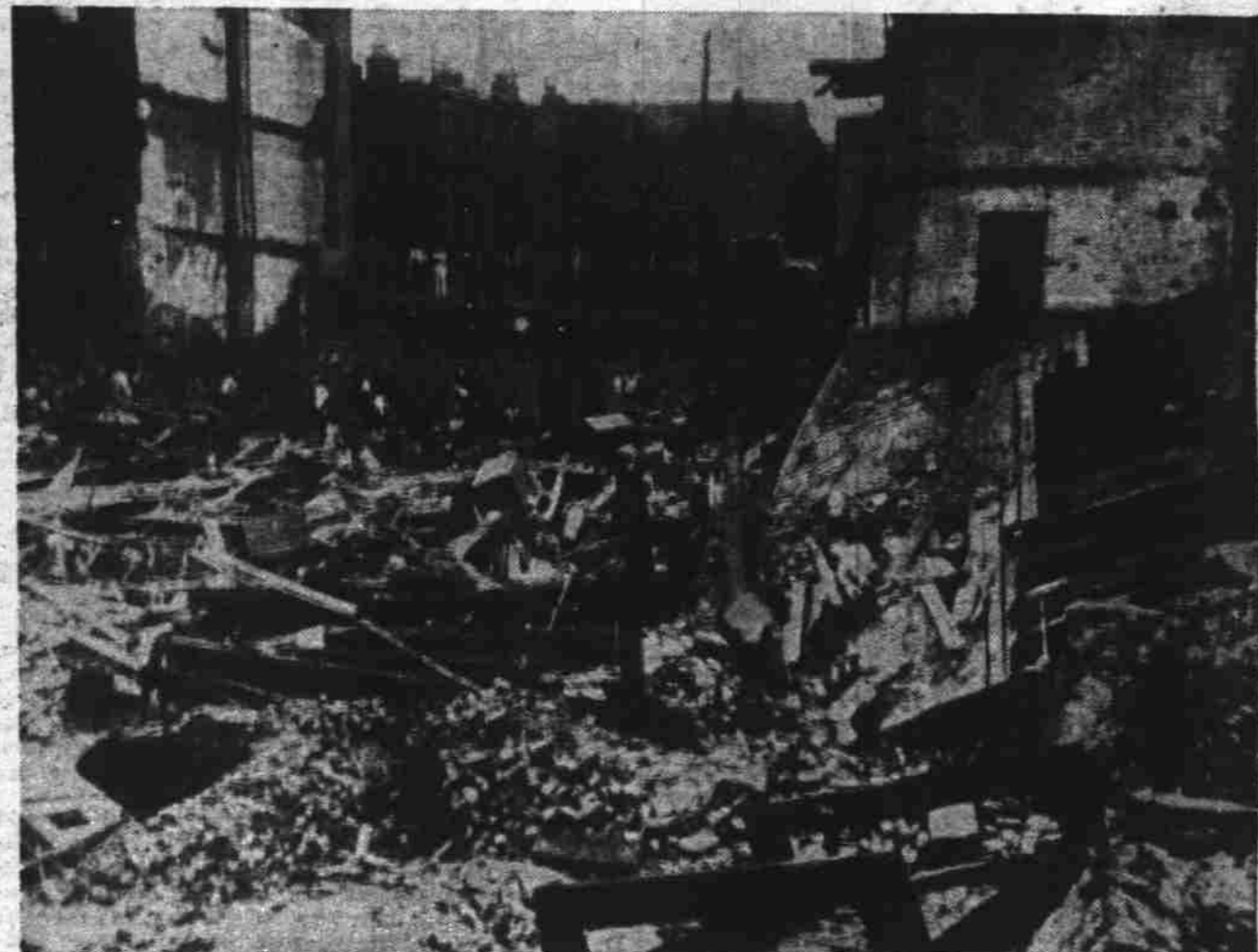
NEW YORK, Aug. 13.—(AP)—Searchers aided by a steam shovel dug deeper today into the mud and splintered timbers of three tenements which collapsed on Staten Island Wednesday night, in search of two more persons missing in the accident that took 19 lives. Nearly all residents of the structure were either unemployed or on relief, Borough President Joseph A. Palma said, appealing for funds to bury them. (Above, view of wreckage.—LIN photo.)
