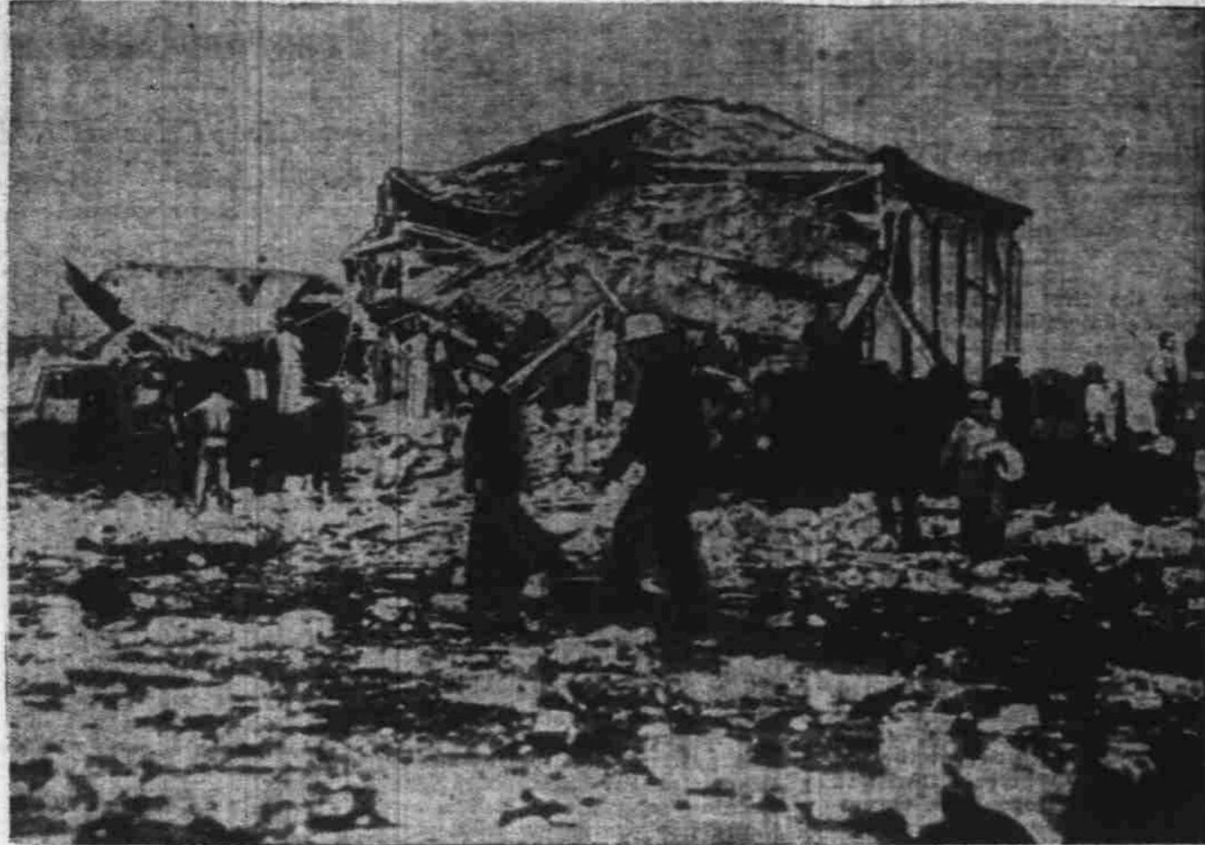
Volunteers from nearby oil fields are pictured as they searched wreckage of the New London, Texas, Consolidated school for the bodies of children who were in the building when it was destroyed by a terrific explosion. This Soundphoto was transmitted directly to San Francisco over telephone wires.
