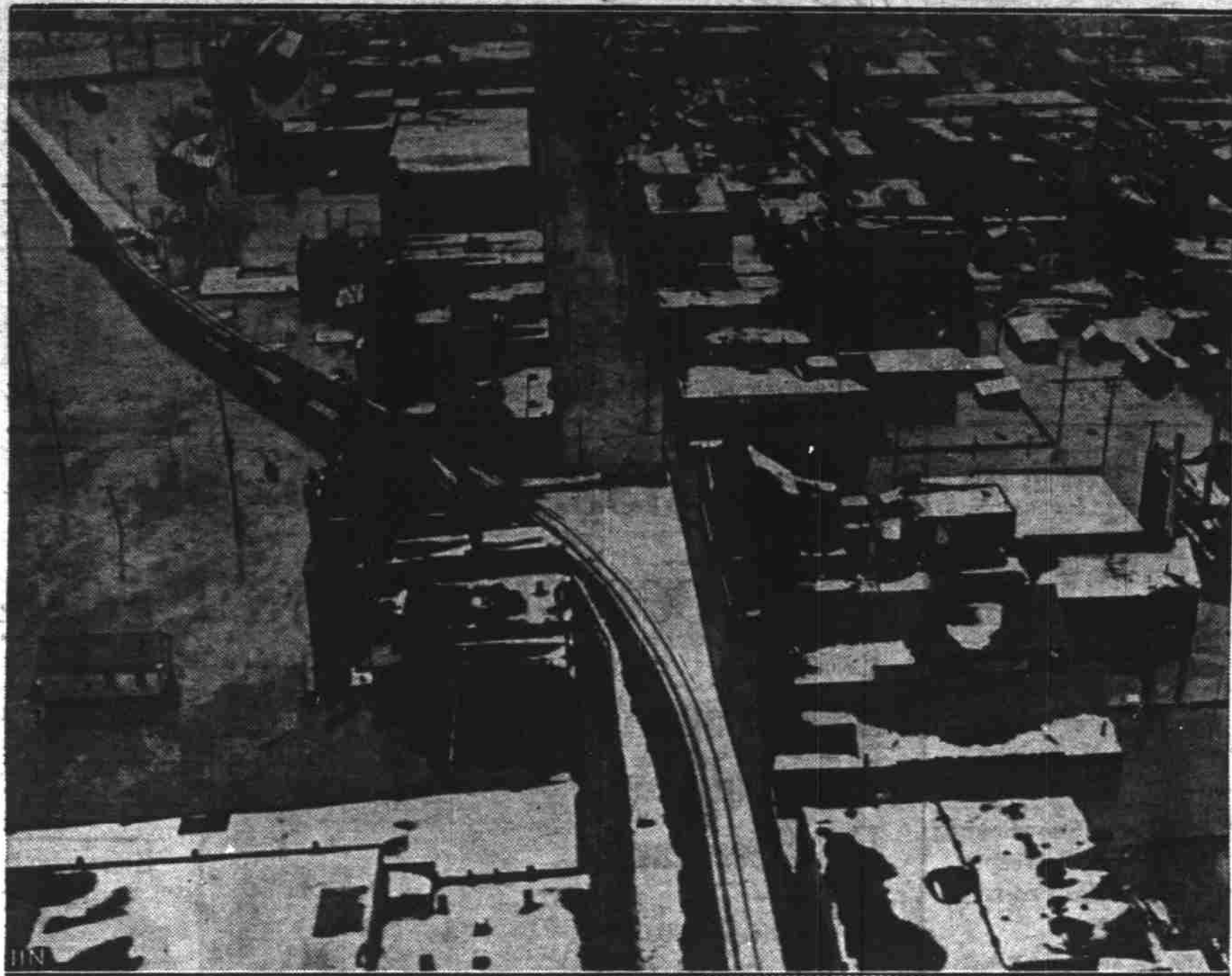
Although this railroad line was elevated at Parkersburg, W. Va., because of the bridge approach, the floods rose to such height that the tracks at each end were under water, preventing traffic from traversing the line.
