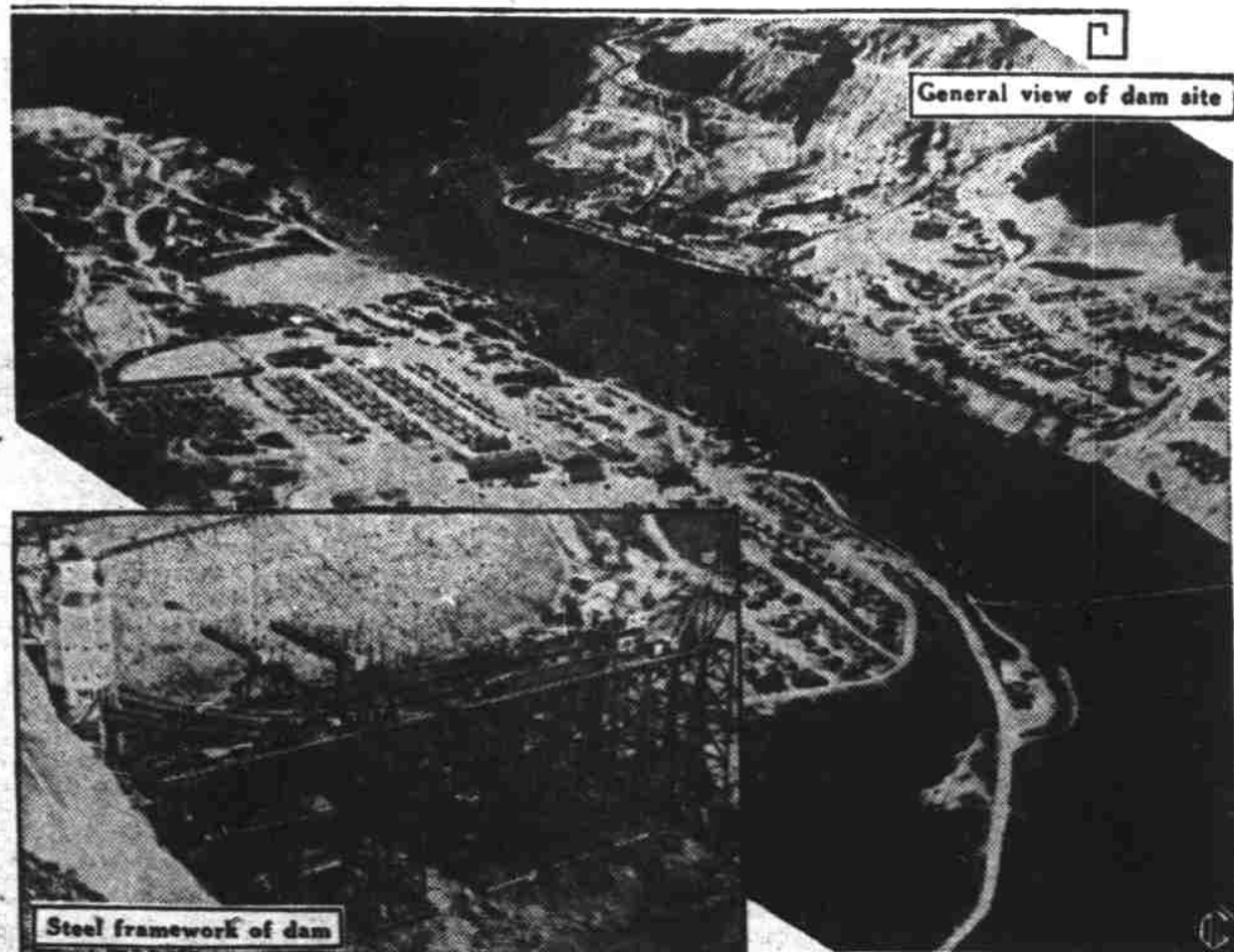
As work progresses on Grand Coulee dam in north central Washington, the largest structure of its kind in the world takes shape, a mass of concrete which will rise to a height of 550 feet above a 500-foot thick base 4,300 feet long over which a
