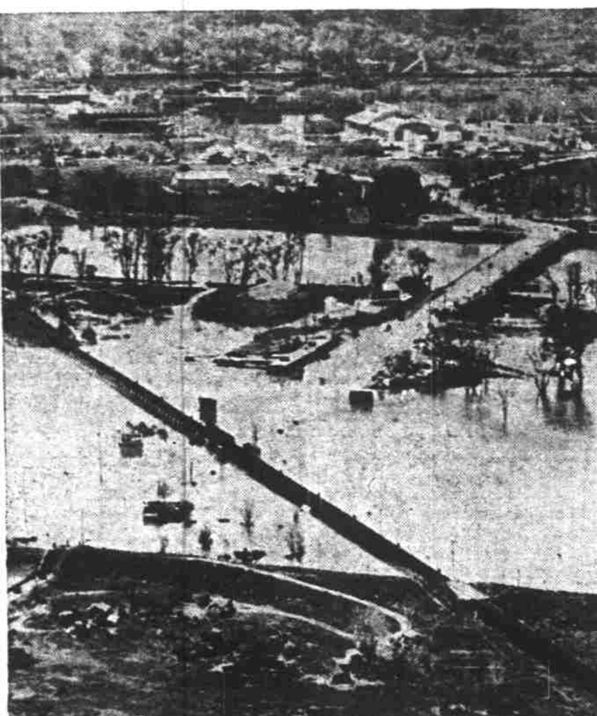
The American river in the Sacramento valley is here shown overflowing its banks, inundating the entrance to the California capital city during the record-breaking flood which followed heavy rains early this week. Twenty-one lives were lost in California due to the storm and flood.—International Illustrated News photo.
