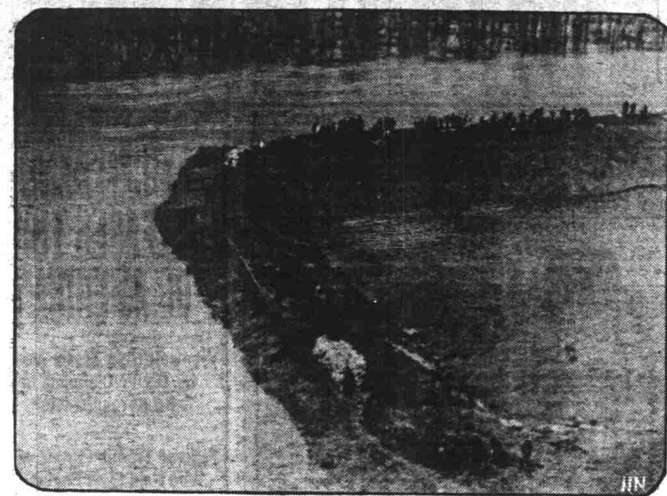
Surrounded by water, flood fighters valiantly struggle to halt the sweep of floodwaters of the Little river, south of Kennett, Mo. The river between levees and trees, pictured above, is 12 feet higher than the water on the other side of the barrier. Observe the sand bags piled on top of embankment.
