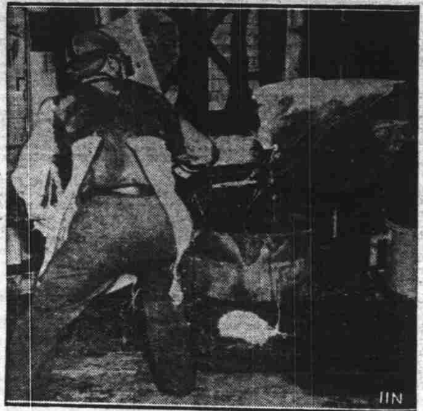
Many noted scientists watched nervously as workers at Corning, N. Y., pour 20 tons of molten glass into the 200-inch telescope mirror mold in a second attempt to make a flawless mirror for the world's largest telescope at Mount Palomar Observatory, California. A year will be required to cool it completely.
