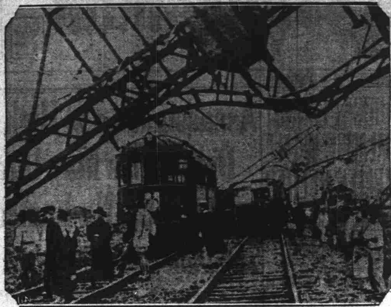
This photo shows a wrecked train and power lines on an express railway line near Tsuruhashi, a suburban station of Osaka, Japan, which were damaged in the terrific typhoon which swept over Japan, leaving in its wake a heavy loss of life and property.
