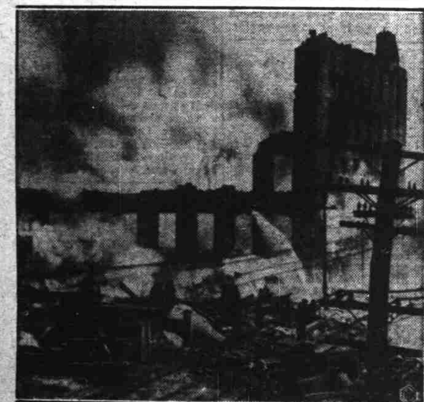
Firemen are shown battling the blaze that did damage estimated at $500,000 at Fall River, Mass. when it destroyed the ancient Merchants Mill, ten other buildings and a gasoline station. A CWA worker was killed and 30 persons hurt as firemen of 12 cities battled flames. Several families were rendered homeless.
