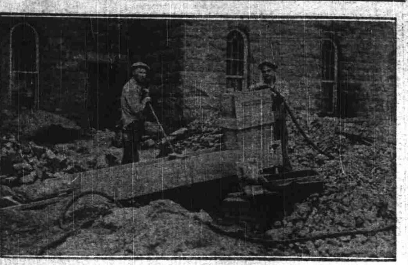
Robert Shiroda is mining in the backyard of the old mint at Carson City, Nev. For many decades sweepings from the floors, ashes from the furnaces and broken graphite crucibles were thrown into the yard. Shiroda, who bought the right to mine the mint grounds to a depth of sixteen feet, for which privilege he paid $100, has employed four miners in the work. Crucibles are broken down with emery wheels to powder in an effort to recover the gold. Shiroda just smiles when asked how the deal is panning out. He is pictured above, at right, with a workman, sluicing waste. International Illustrated News photo.
