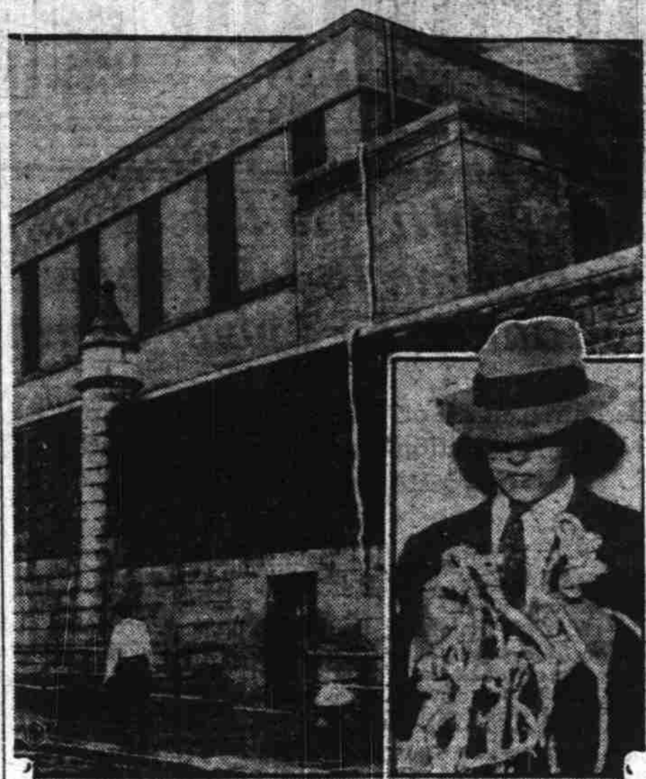
Here is the spot at New York's historic Tombs Prison wall where three convicts made a smooth, bloodless escape via the improvised rope shown hanging from the roof. The rope, shown in hands of investigator (inset), was fastened from sheets hung with wire from bedsprings. The fugitives, James McNally, Henry Simmons and Gerard Simonson, were waiting trial on charges of burglary and gun-toting.
