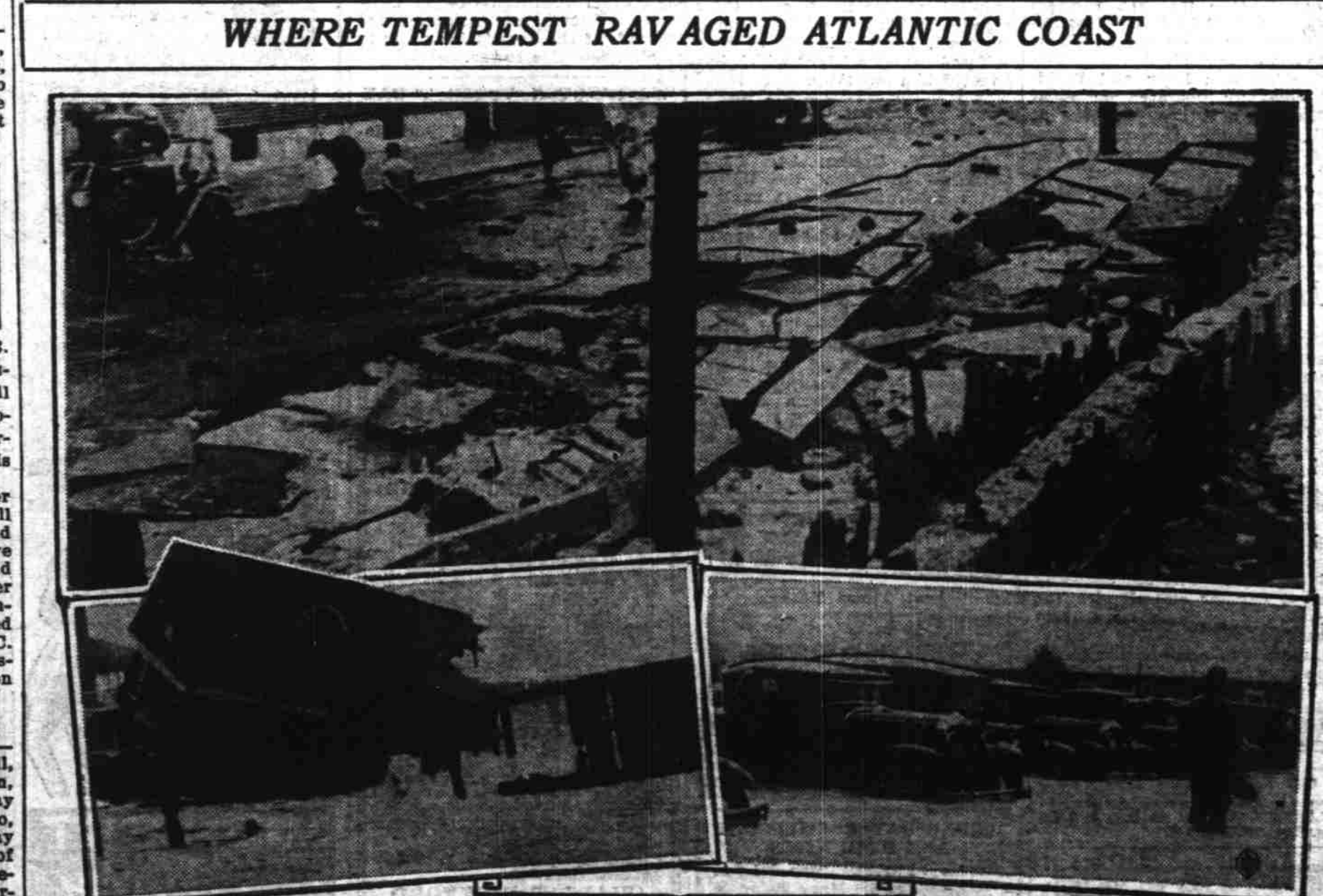
These pictures tell a graphic story of the savagery with which the terrific hurricane lashed the Atlantic coast, causing untold damage to property. Top photo shows the heavy concrete road along the sea wall at Atlantic City, N. J., reduced to battered fragments by the pounding of mountainous seas. Lower left, a one-story house at Seabright, N. J., undermined by the waves and smashed beyond repair, and lower right, a few of the hundreds of automobiles abandoned by their owners at Wilmington, Del., when gale-whipped waves flooded the city.
