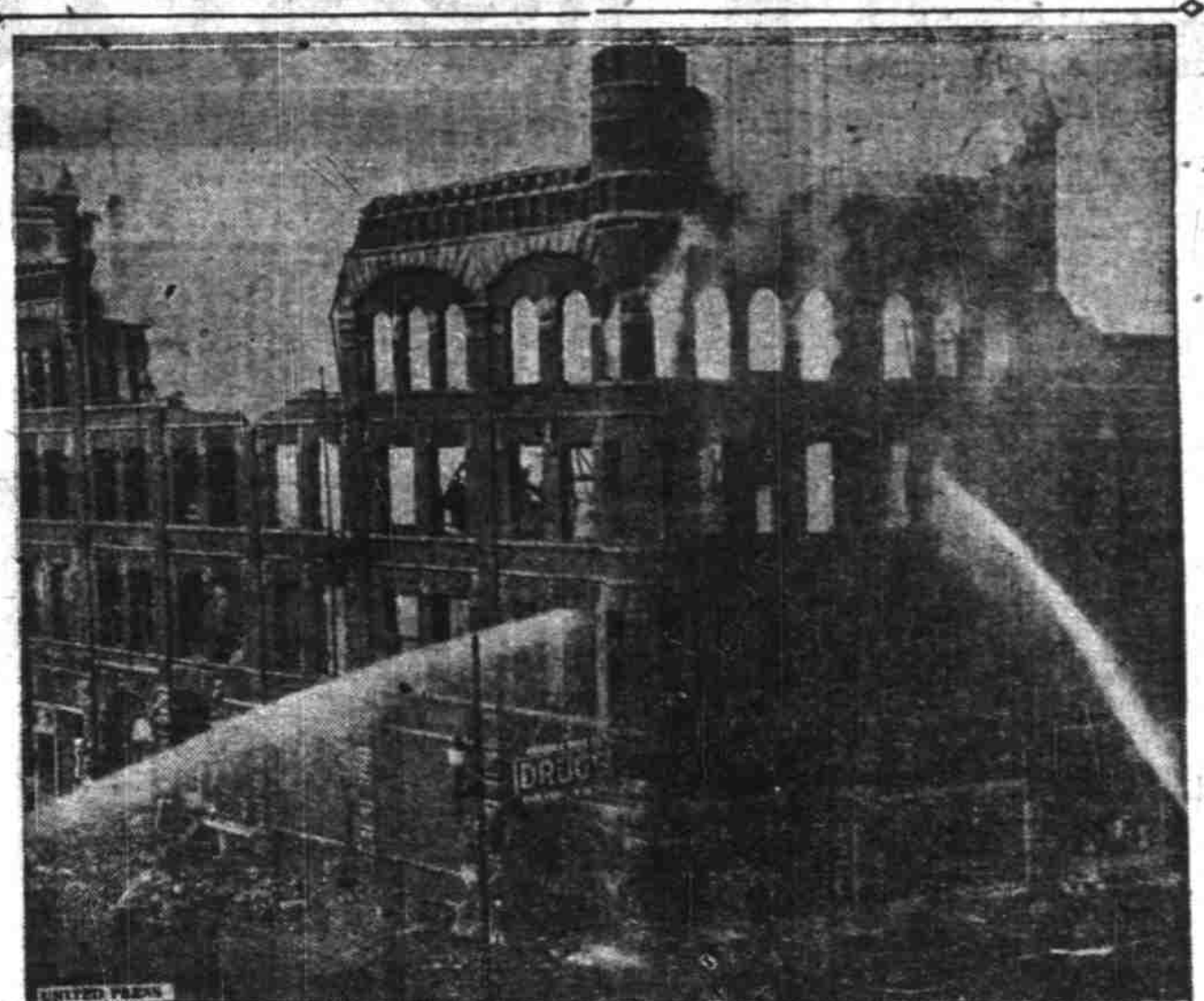
National fire prevention week had no sooner dawned than two of Montana's largest business block fires got underway. This photo shows the Hammond Block in Missoula, being gutted by flames. Seven business establishments were destroyed and 40 occupants of apartments were driven to the street in smoky attire. At the same time a similar fire occurred in Butte, raising a building which contained four business houses and two hotels. Thirty-five persons were forced to flee to the ice-covered streets. Total damage of approximately $500,000 resulted from the two fires.
