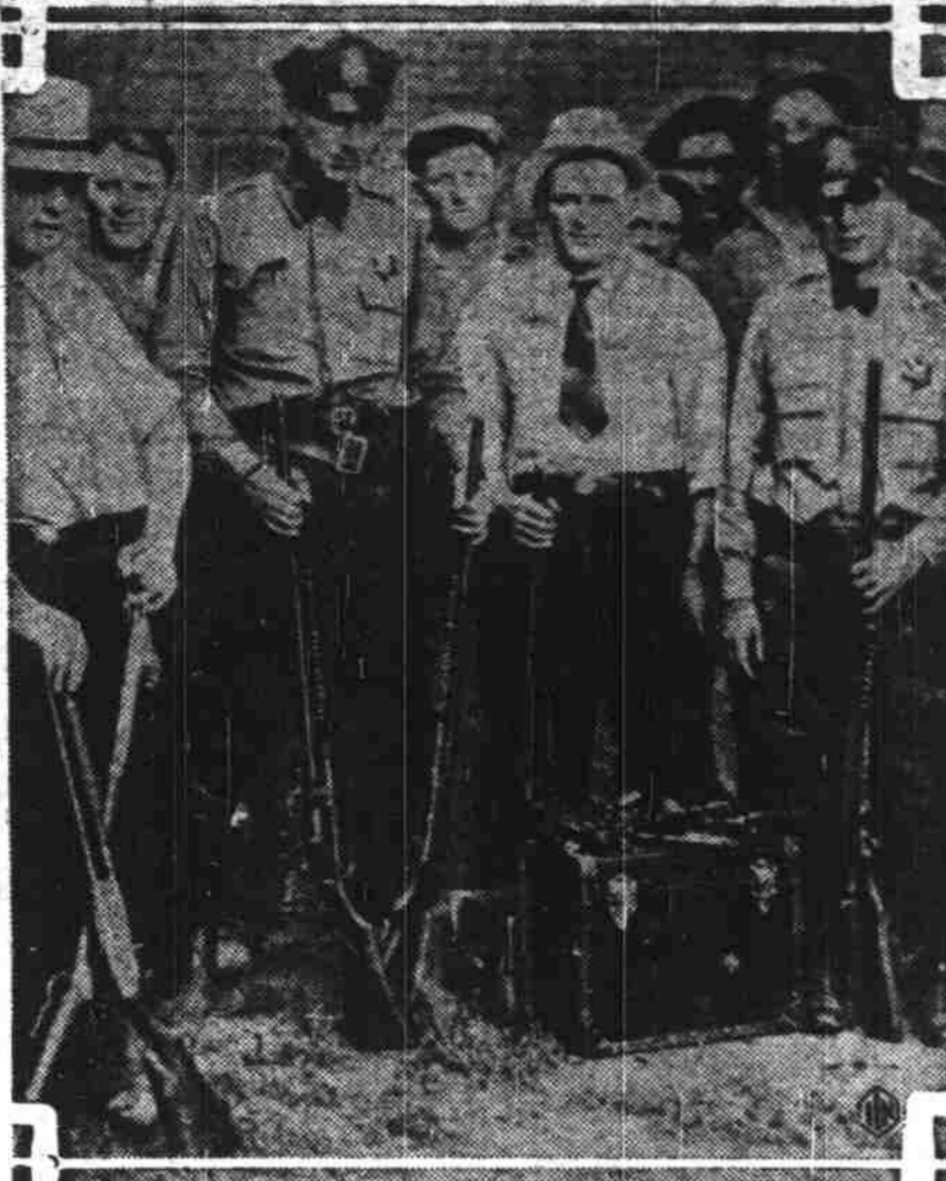
Following a labor riot in which one man was killed and over a score injured, these heavily armed guards and State Police are protecting the workers on the cofferdam being constructed on the Illinois River, near Marietta, Ill. The labor union claims that the companies doing the work are paying far below union wages and that they are also importing cheap labor from other States, keeping union men out of work.
