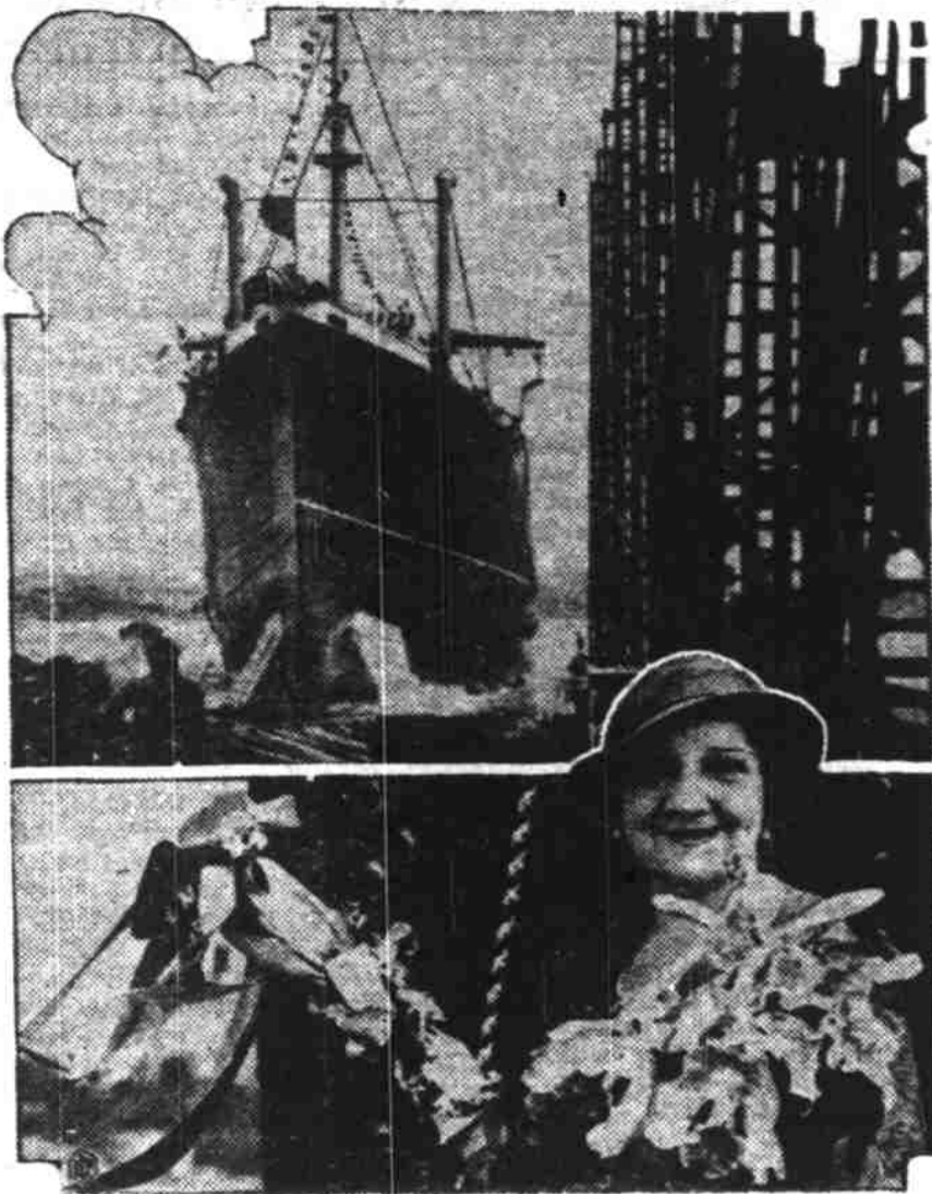
A good job well done, and the new $5,000,000 Grace liner, Santa Paula, slides down the ways and into the water at Kearney, N. J., to the cheers of the workmen who built her and officials of the line. Lower photo shows Mrs. Edward J. Ford, wife of the president of the Panama Mail Service of the Grace Line, as she broke a bottle of California orange juice on the bow of the new vessel during the christening ceremonies.
