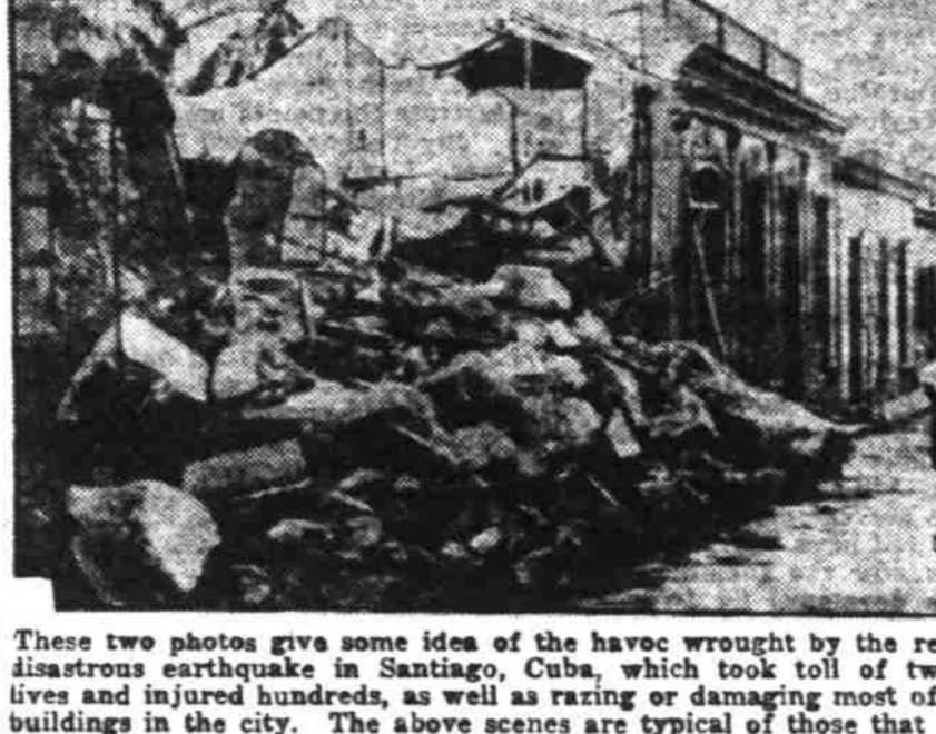
These two photos give some idea of the havoc wrought by the recent disastrous earthquake in Santiago, Cuba, which took toll of twelve lives and injured hundreds, as well as razing or damaging most of the buildings in the city. The above scenes are typical of those that prevail in almost every street in the former capital of Cuba. Though the first severe shock lasted only 30 seconds, it damaged buildings so badly that succeeding minor shocks completed the work of destruction.
