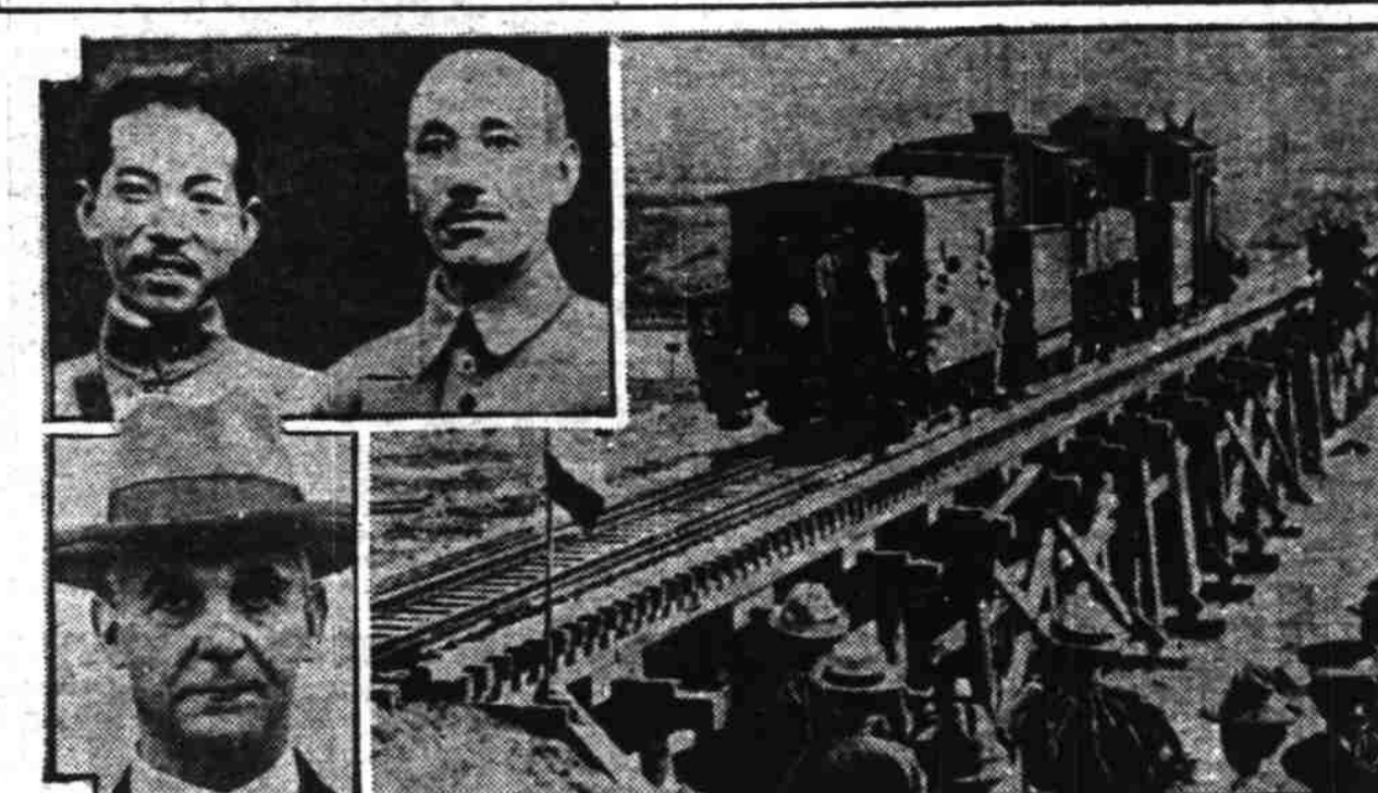
The Kiangching river railway bridge of the Tsaoan-Anghachi line, following its repair by the Japanese forces now in Manchuria, since the Chinese soldiers and engineers had failed to fix it. The first engine to cross the bridge since its destruction is shown. The repair of the span cost 250 lives, what with Chinese firing on the Nippon repair gang and Japanese troops retreating on the Chinese. In upper left, Marshal Chang Hsueh-Liang (left) deposed Manchurian governor, and President Chiang Kai-Shek, the national leader, are depicted. General Charles F. Sumnerall (lower left), retired, former United States chief of staff, may lead the international commission which the League of Nations is suggesting as a solution of the Manchurian crisis.
