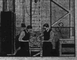
The Impact Test A heavy steel ball is dropped sixteen feet on the glass used for the Ford windshield as an impact test. Even under this severe blow there is no flying glass.
