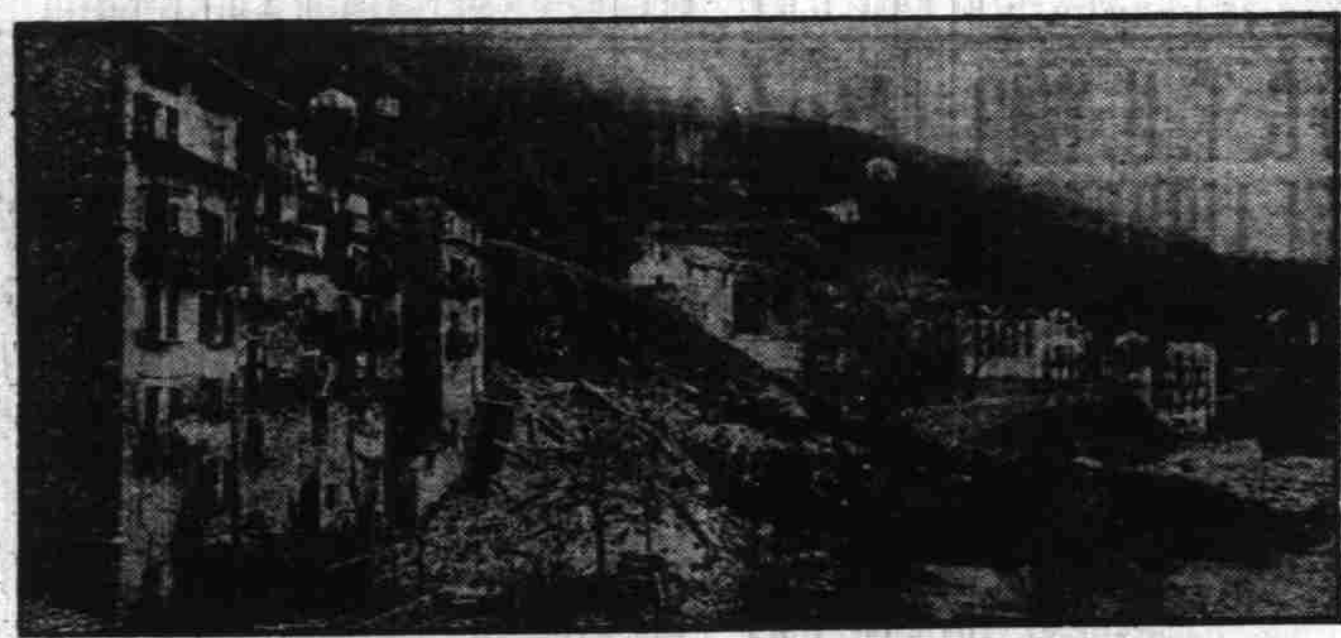
Three landslides occurred in succession, engulfing houses in the fair city of Lyons, France, where authorities say at least seventy persons were killed.
