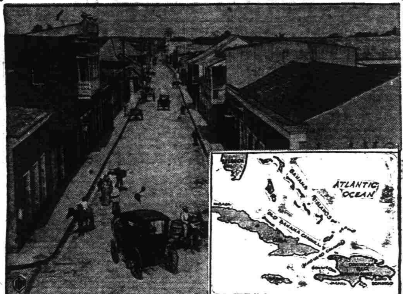
Peaceful street scene in Santo Domingo City, the capital of the Dominican republic, situated on the Island of Haiti, now in the grip of a 136 mile per hour hurricane. The city has been cut off from the outside world by the storm, making it impossible at this time to compute loss of life and property damage. (Inset) Map shows the Dominican republic of 38,000
