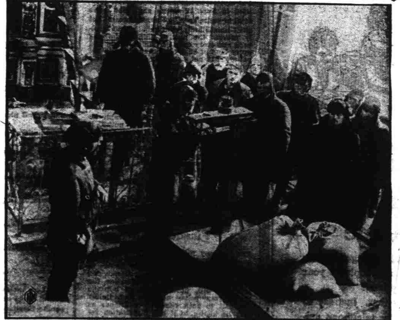
Churches and monasteries are being demolished in Russia in the Soviet's mad rush toward atheism. Below, some mellow tones have called the faithful to worship for centuries, are being crushed from their towers and melted so that the metal can be used for the manufacture of farm implements. The churches have been converted into granaries in the Soviet's new craze for "culture." Picture shows peasants of Petrovsky village bringing their wheat to a church which has been transformed into a granary.
