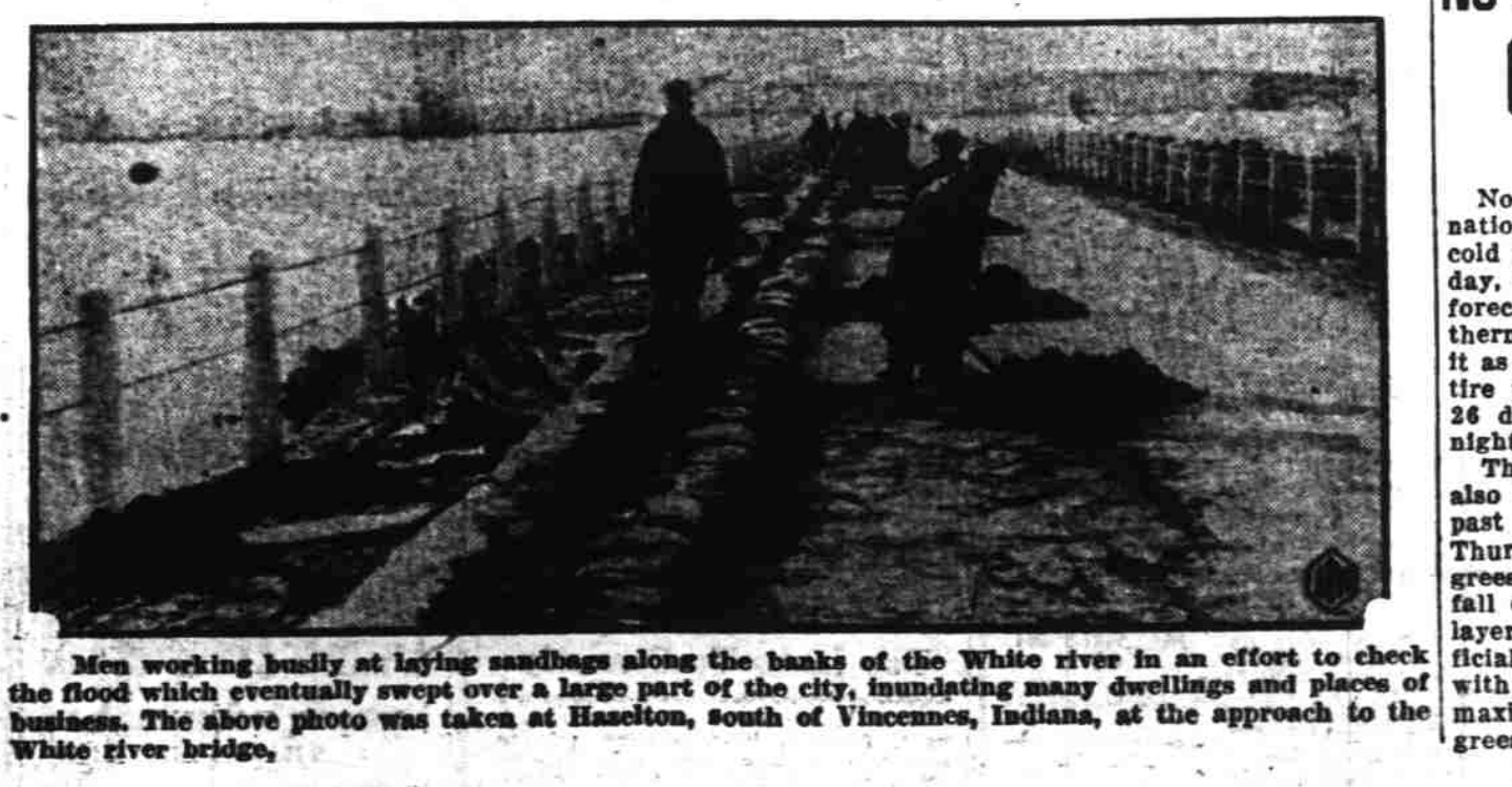
Men working busily at laying sandbags along the banks of the White river in an effort to check the flood which eventually swept over a large part of the city, inundating many dwellings and places of business. The above photo was taken at Hazelton, south of Vincennes, Indiana, at the approach to the White river bridge.
