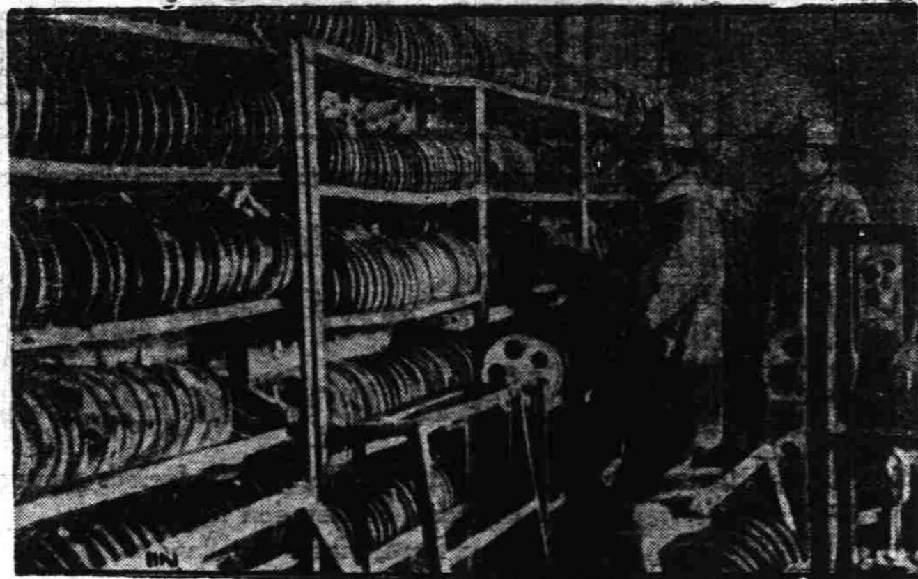
Captain E. W. Nast and J. C. Wist, of the Hollywood Fire Department, inspecting rolls of film in the laboratory of the Consolidated Film Industries, at Hollywood, Calif., following the explosion and fire which caused an estimated damage of $50,000,000 and loss of one life. The bulk of the loss lies in the destruction of the countless rolls of master negative feature films which cannot be replaced. The building itself was only valued at $400,000.
