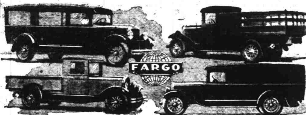
Here are four body styles of the "Freighter", new product of the Fargo Motor Corporation, truck division of Chrysler. The Freighter has a wheelbase of 133 inches and is powered by a 55 h. p. Chrysler six-cylinder engine. Fargo has been building 3/4 and 1/2 ton delivery equipment for eight months. The "Freighter" has just been added to the line.
