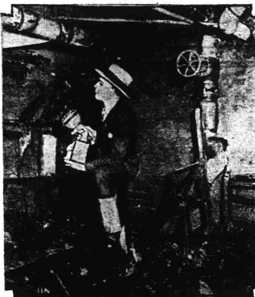
With a death toll of 14 lives, the investigations into the Cleveland Clinic hospital fire are tending to show that the explosion was caused by over-heating of X-ray films stored in the room above. Modern safeguarding apparatus, constructed to function when exposed to heat, failed to act, allowing the gas set off by the burning films to spread through the hospital.
