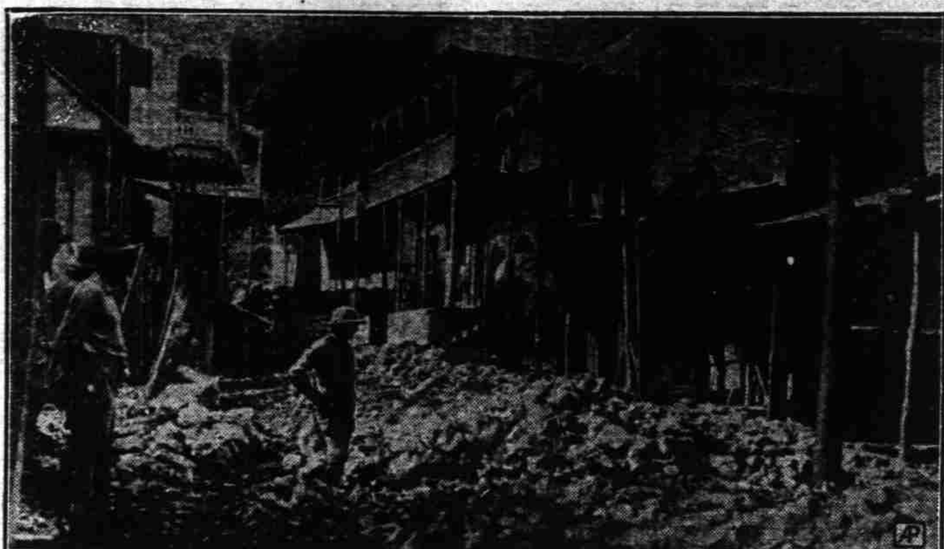
MAJOR DESTRUCTION OF BUILDINGS, BRICKS, PLASTER AND OTHER MATERIALS WHICH OVERLOOKS A LARGE AREA, KILLING ANIMALS AND DESTROYING CROPS AND FOOD SUPPLIES. RELIEF WORKERS ESTIMATE THAT 100,000 ARE FACING FAMINE IN THE STRICKEN AREA.
