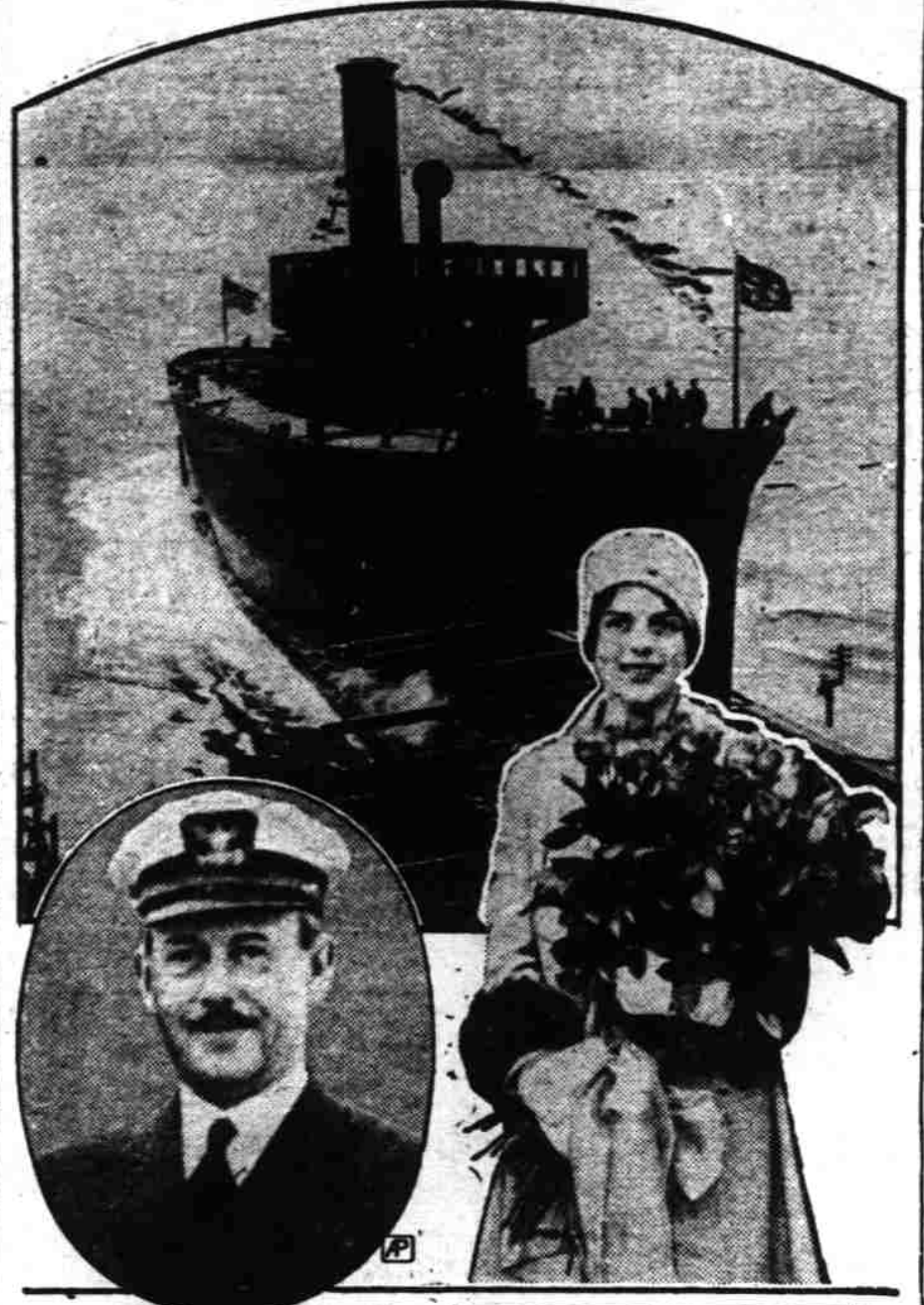
The Coast Guard Cutter Pontchartrain, one of five modern vessels soon to join the fleet, takes the water at the Fore River Shipyard, Quincy, Mass. Mrs. Newton Gifford of Fall River, Mass., (right) christened the craft and Comm. F. A. Hunnewell designed it.
