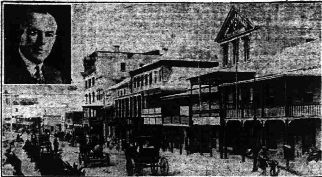
E. T. Strong, president of the Buick Motor Company, found plenty wrong with it, from an automobile maker's standpoint, when he visited the place recently. For this photo was taken in Bermuda, which has motor cars, and this street scene is typical of hundreds of others on that island. Many of the residents here have
