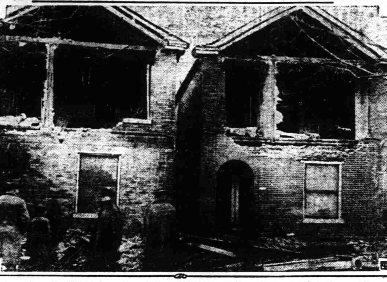
Scenes from the districts in southern Ohio and Kentucky hit by cyclonic winds, which caused heavy damage and many injuries. Above, a street scene in Hamilton, O., where damage was reported heavy. Below, wrecked buildings on Southern Parkway, in Louisville, Ky., which also suffered heavy damage.
