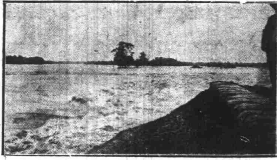
Mississippi river pouring through a crevasse at Melville, La., 30 minutes after the dyke gave way to the flood.
