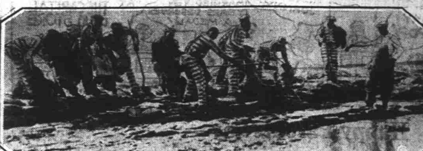
Unusual photo of convicts at Little Rock, Ark., vainly trying to stave off flood in the Arkansas river by packing sandbags in the gum soil
