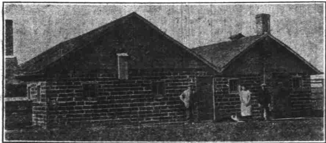
The hollow tile, double incubator house of Lloyd A. Lee. Since the above picture was taken a large addition of similar construction has been built on the building at the right. Mr. and Mrs. Lee and their incubator expert, Mr. Armstrong, are shown in the picture.
