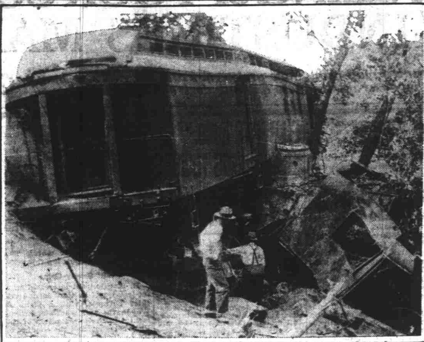
A broken locomotive wheel resulted in the derailment of a Louisville & Nashville train near Canton, Ga., and brought about the deaths of the engineer and fireman. The passenger coaches miraculously escaped serious injury. The illustration shows the baggage car, which plunged down an embankment on top of the derailed engine.
