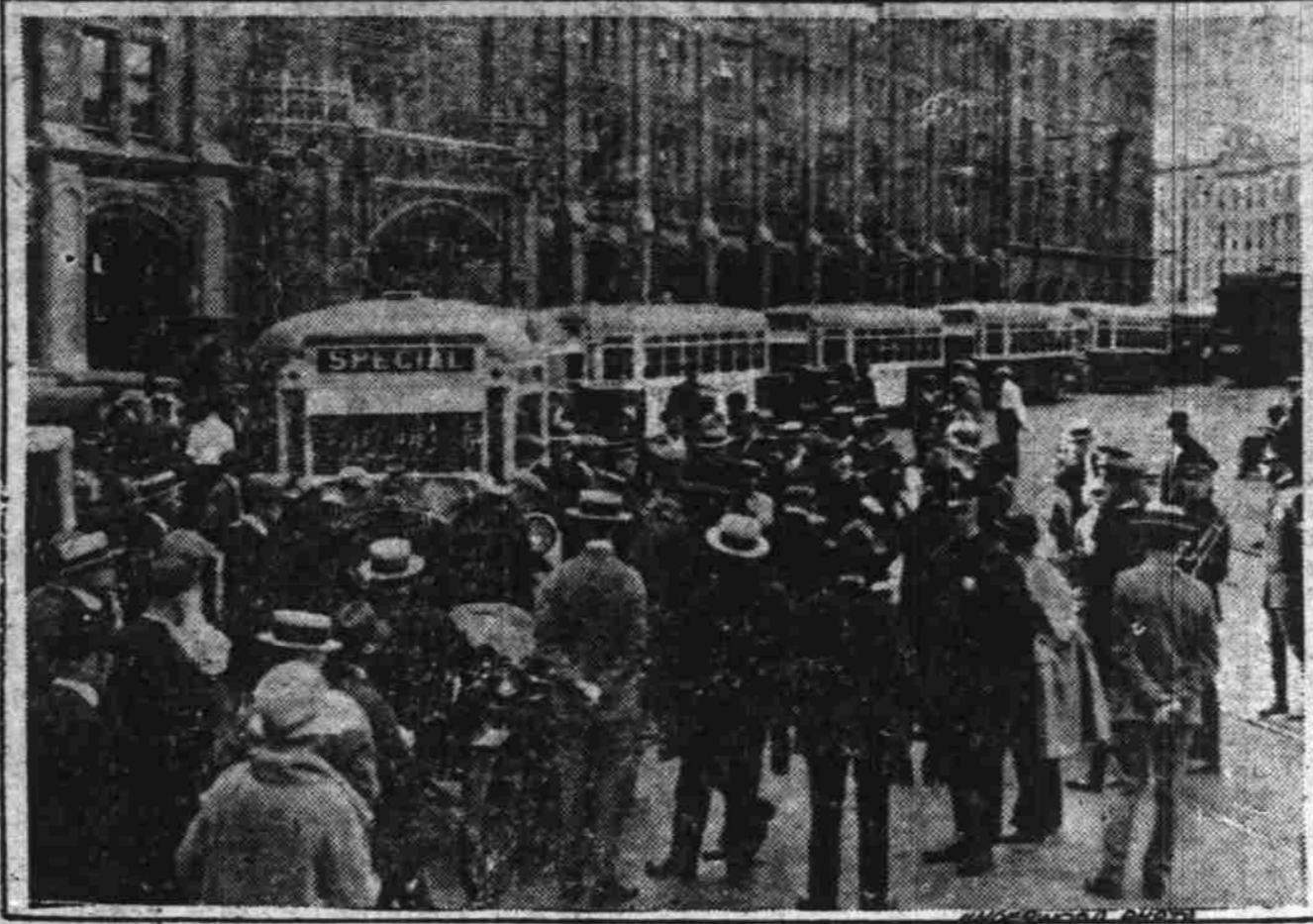
The street railway company in Albany, N. Y., is supplanting its cars with busses, the first company, it is said, to voluntarily do so. A fleet of the busses is seen taking over a tram line. Busses are making such enormous inroads into the business of electric railways that many authorities see the industry as doomed. Others disagree, and say the traffic problem will bring the electric car back.
