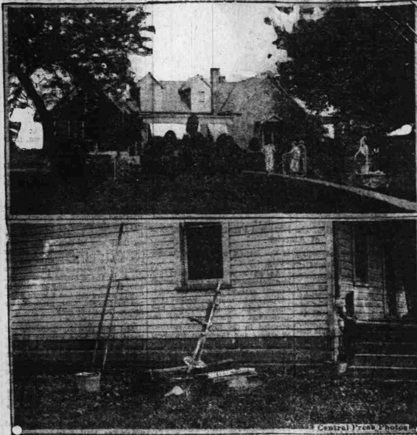
Above: The Thomas seaman residence; below, the cistern.
