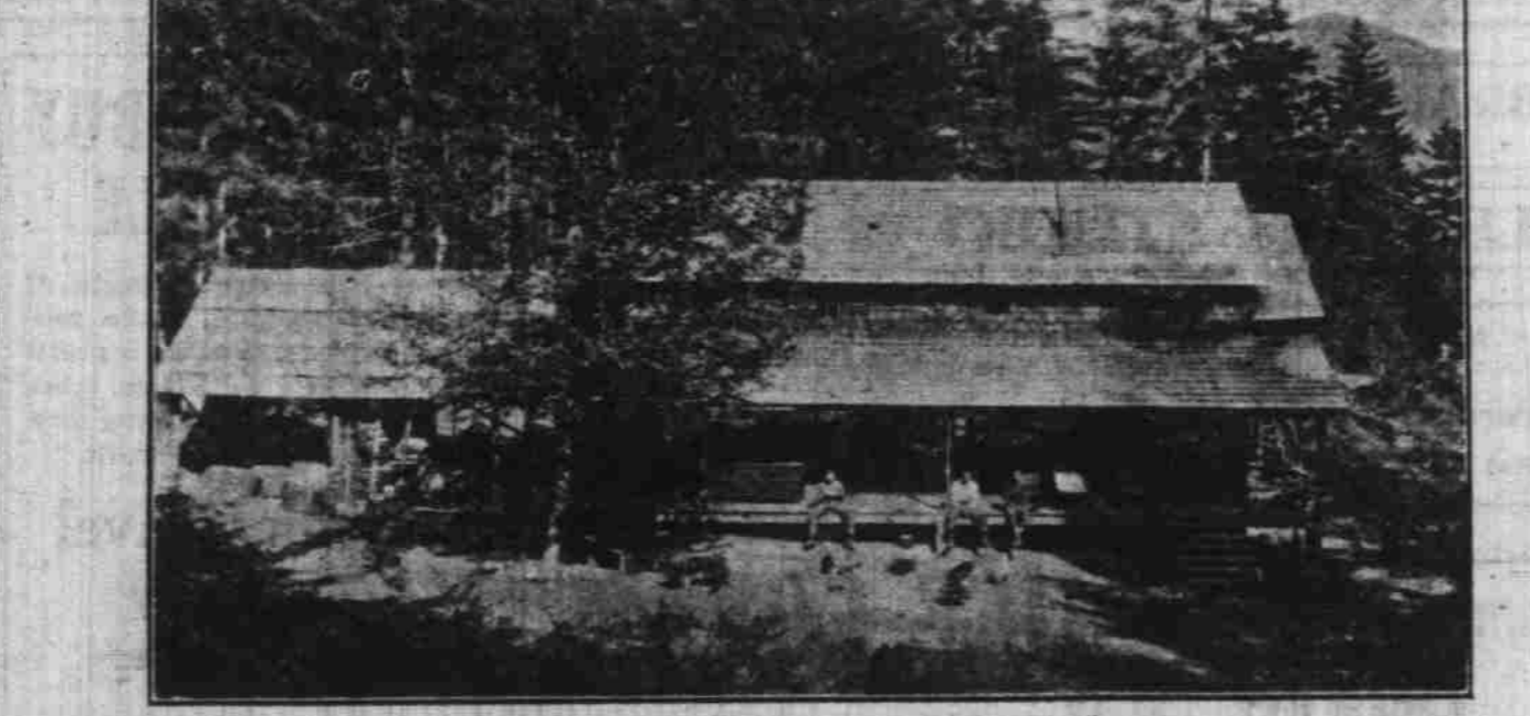
Camp at Silver King Mine
