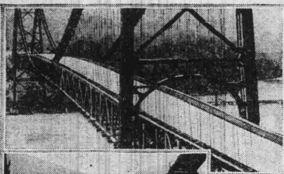
The New Hudson River Bridge at Bear Mountain now open. Last work was laying of a 38-foot wide asphalt roadway.
