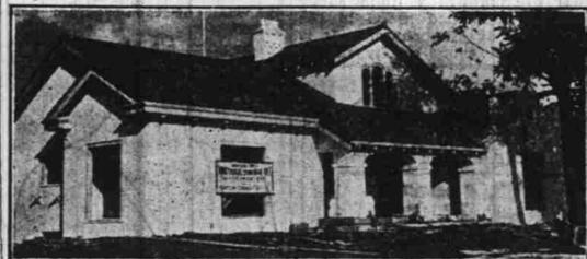
Distinctive new stucco and tile roof residence of B. E. Edwards nearing completion at 19th and State streets of this city. This home was erected by G. M. Douglass, interior and exterior finish by R. Ritacca, and roofed with red "Water-seal" concrete roof tile manufactured and laid by the Oregon Gravel Company.
