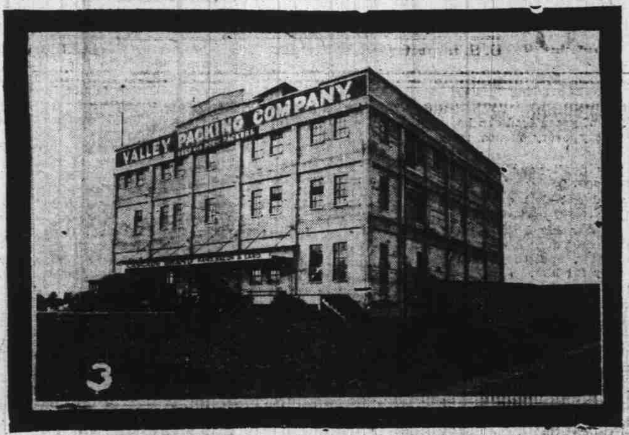
A view of the Valley Packing company plant, first unit, taken several years ago. It appears much enlarged and improved now, and a new photograph will be taken soon, and a new cut made, when all the finishing touches are put upon the main building with its additions.
