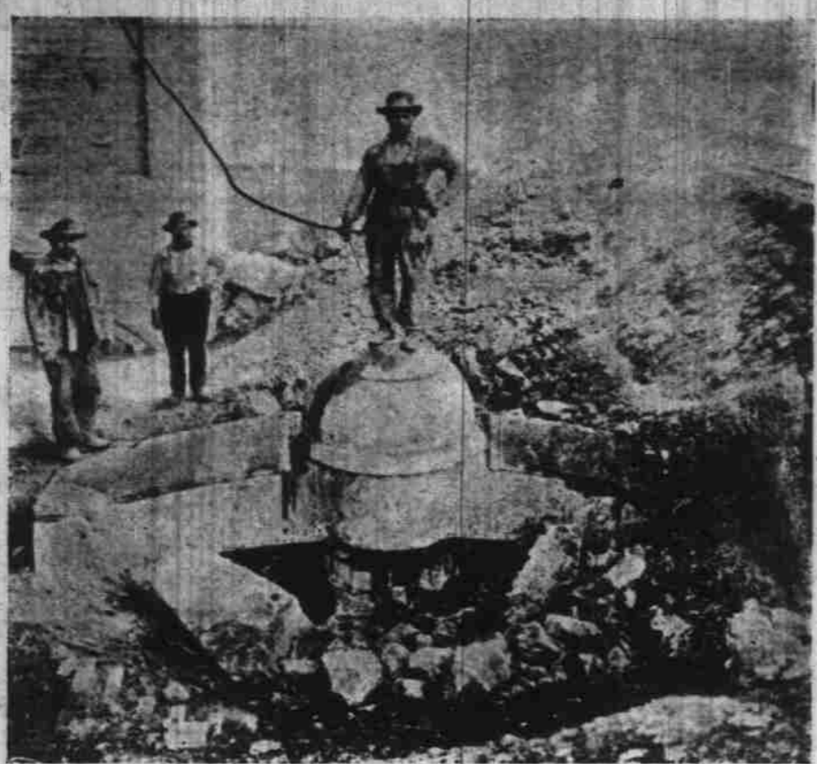
A gyratory crusher used in the cement mills. The huge pieces of stone as they come from the quarry are first crushed in a machine like this.
