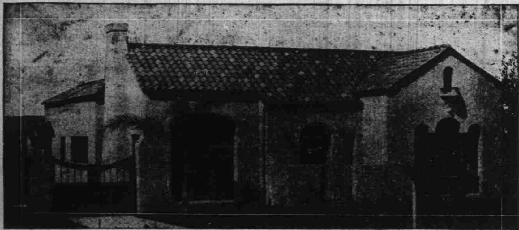
A California Mission Style Bungalow, constructed of Burned Clay Hollow Building Tile and covered with a Light Buff Stucco. The roof is Mission Style Burned Clay Roofing Tile
