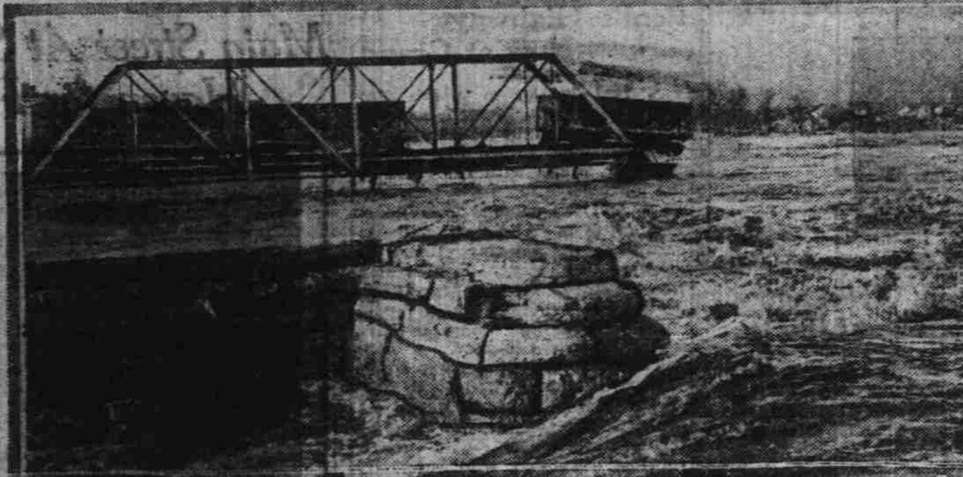
Heavy rains were caused in the Potomac when the river rose twenty feet above its normal level. This photograph shows the wreckage of the Western Railroad bridge near Hancock, Md. after the flood, waters had torn it from its foundations.
