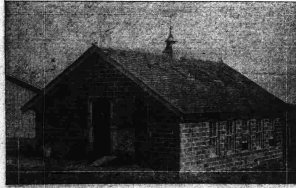
Gable roof type poultry house of hollow building tile.
