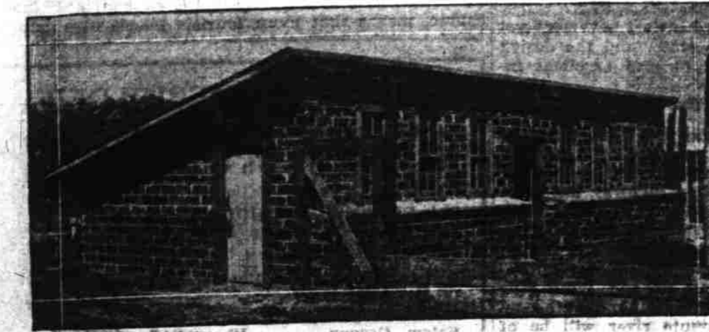
Shed roof type poultry house of hollow building tile
