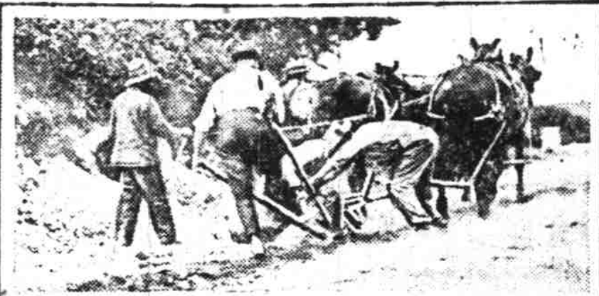
Plowing To Make a Road
