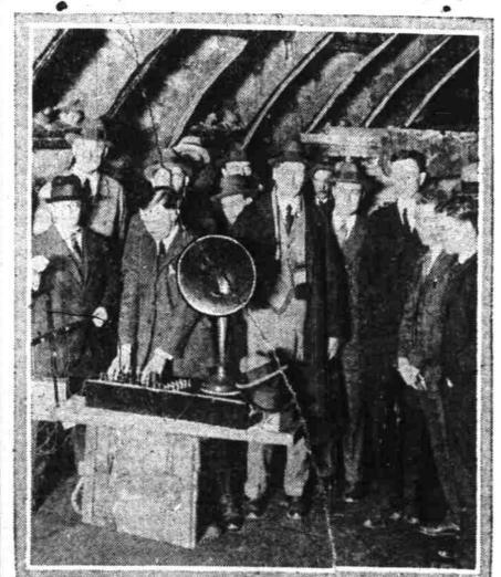
Experiments in radio broadcasting were recently conducted to determine whether the waves would penetrate through the New York-New Jersey vehicle tunnel now being constructed under the Hudson River. Broadcasting was distinctly heard through 500 miles of air, 70 feet of water, 30 feet of much and the heavy steel casing of the tunnel. Photo shows a receiving set in the steel tunnel seventy feet under water.
