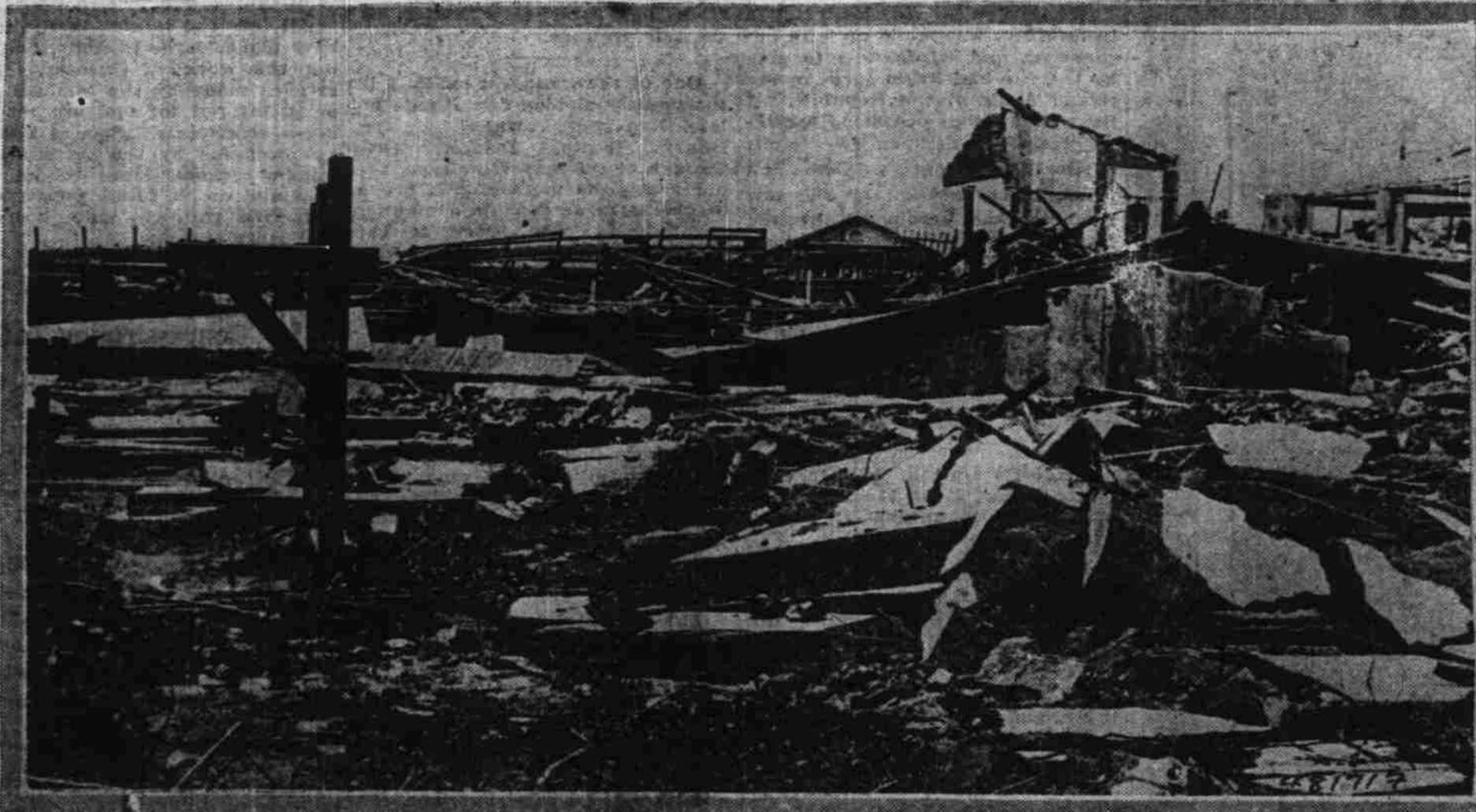
Photo shows view of the jumbled mass of ruins left in the wake of the earthquake and tidal wave at Yokohama.
